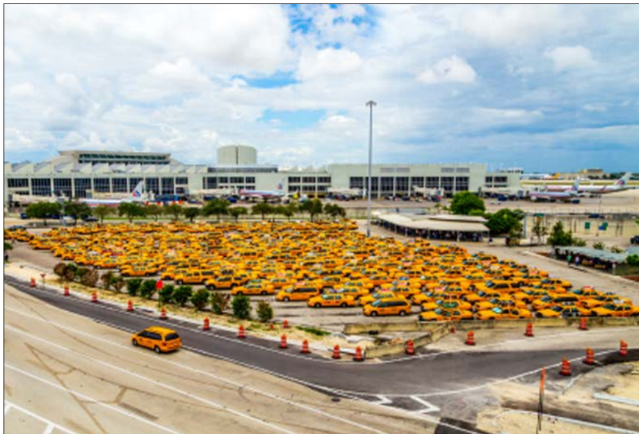
Miami International Airport has been working on several renovation projects as part of their $6.4 billion Capital Improvement Program in 2011.
